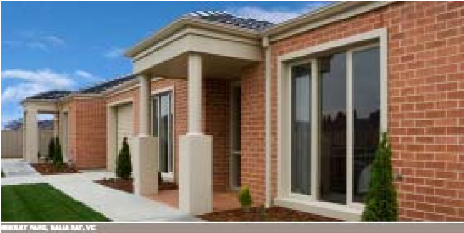
WINDLEY PARK, FALLA HAV, VA
